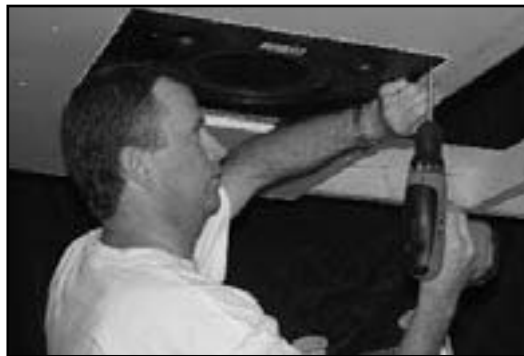
Figure 8: Attaching the subwoofer to the PIR.
